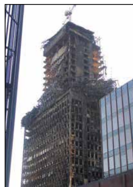
Figura 10.9. Torre Windsor. Madrid.
